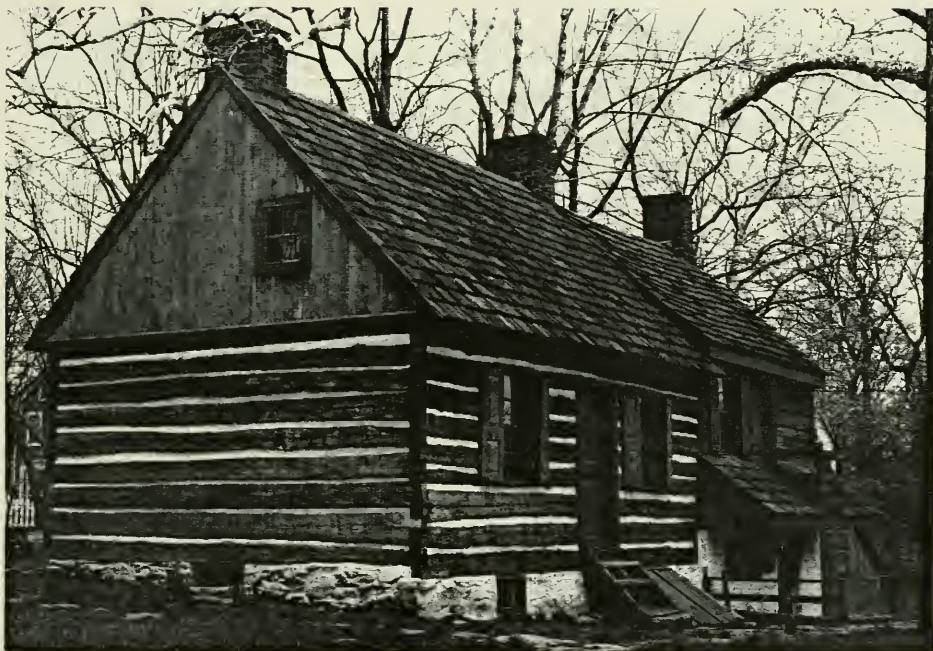
Fallsington - Moon-Williamson Log House, front facade
